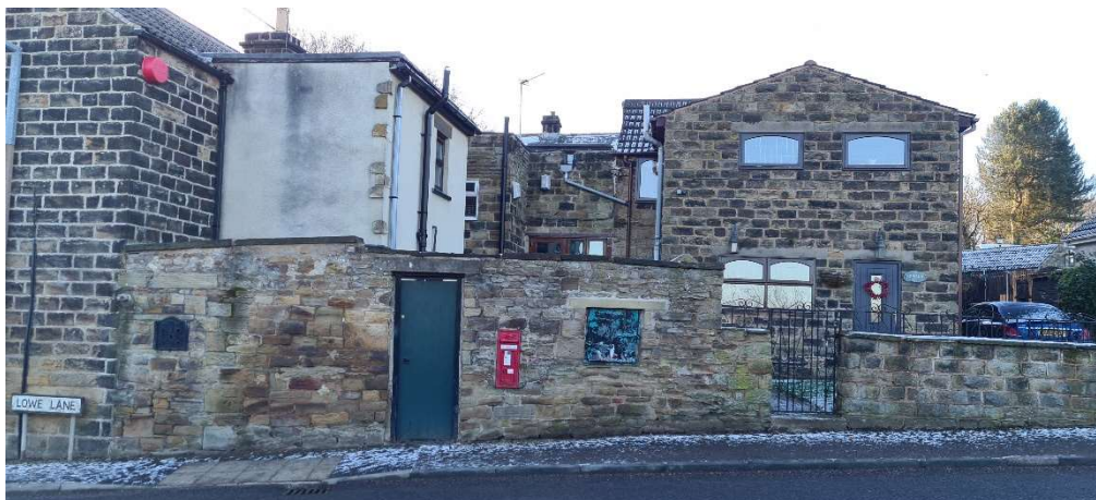
FIG 3. PHOTO : FRONT ELEVATION LOWE LANE
