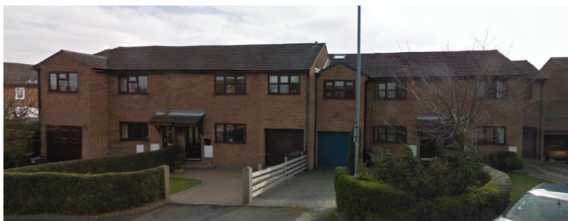
Two houses have been considerably extended and joined
