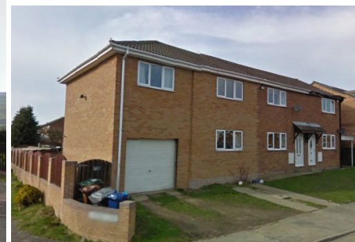
First building on Copster Close west side has been extended by over twice its original length with no step in roof or façade.
