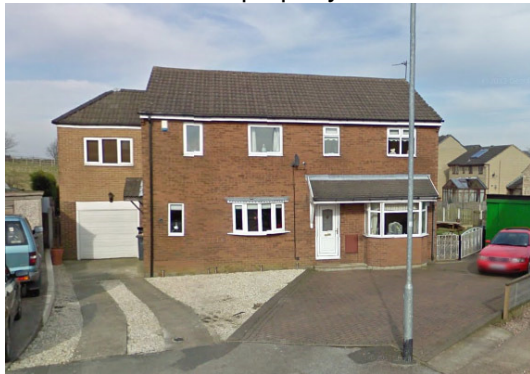
A stepped extension with hipped roof
