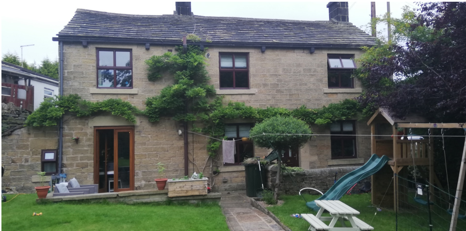
East elevation and garden
