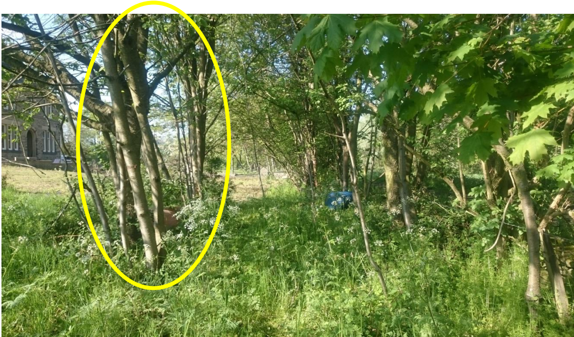
Photo 5. Showing trees 028 to 030 that are to be removed, along with various saplings (sucker growth) in the same row. Only those trees within yellow circle are to be removed – screening from the track remains on the right of picture.
