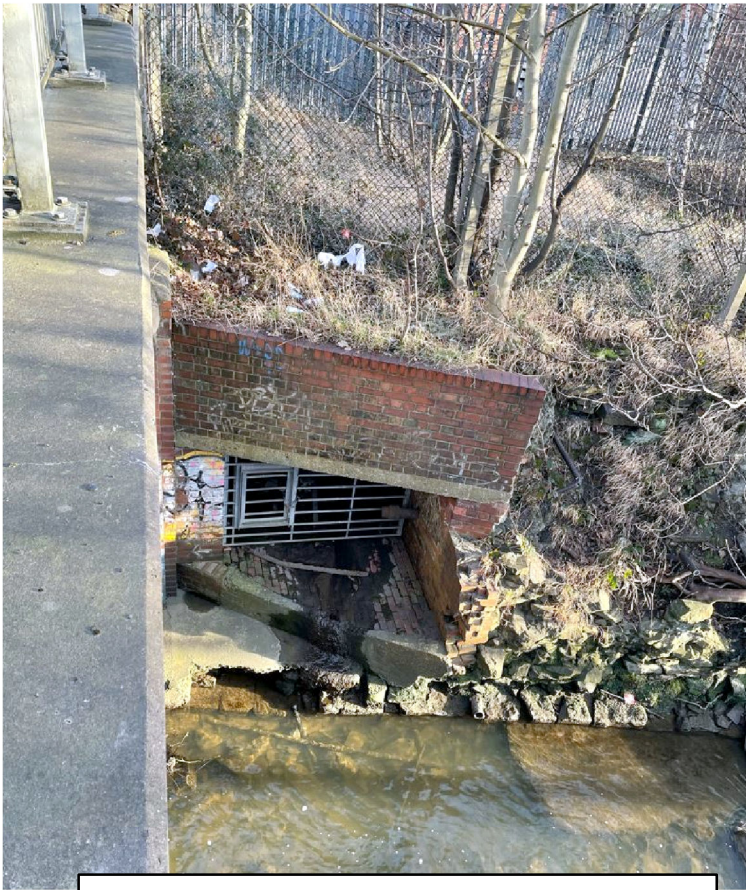
Culvert entrance viewed from Old Mill Lane Bridge.
