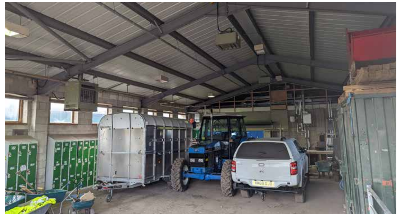
Photograph of interior of Tractor Shed from main access door
