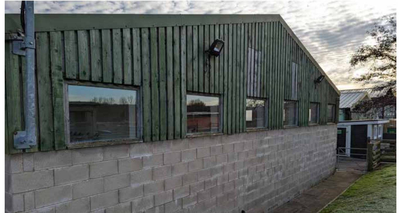
Photograph of West Elevation of existing Tractor Shed from north west
