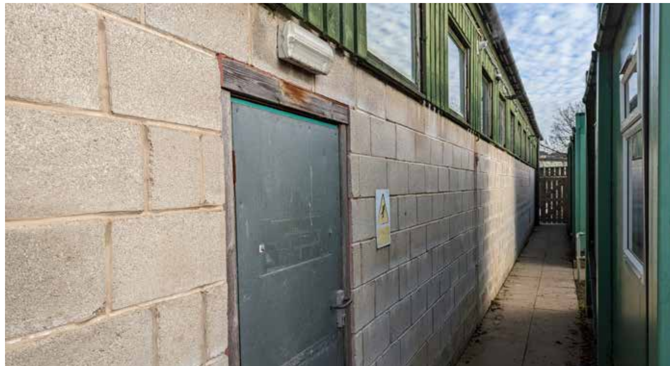
Photograph of South Elevation of existing Tractor Shed from west
