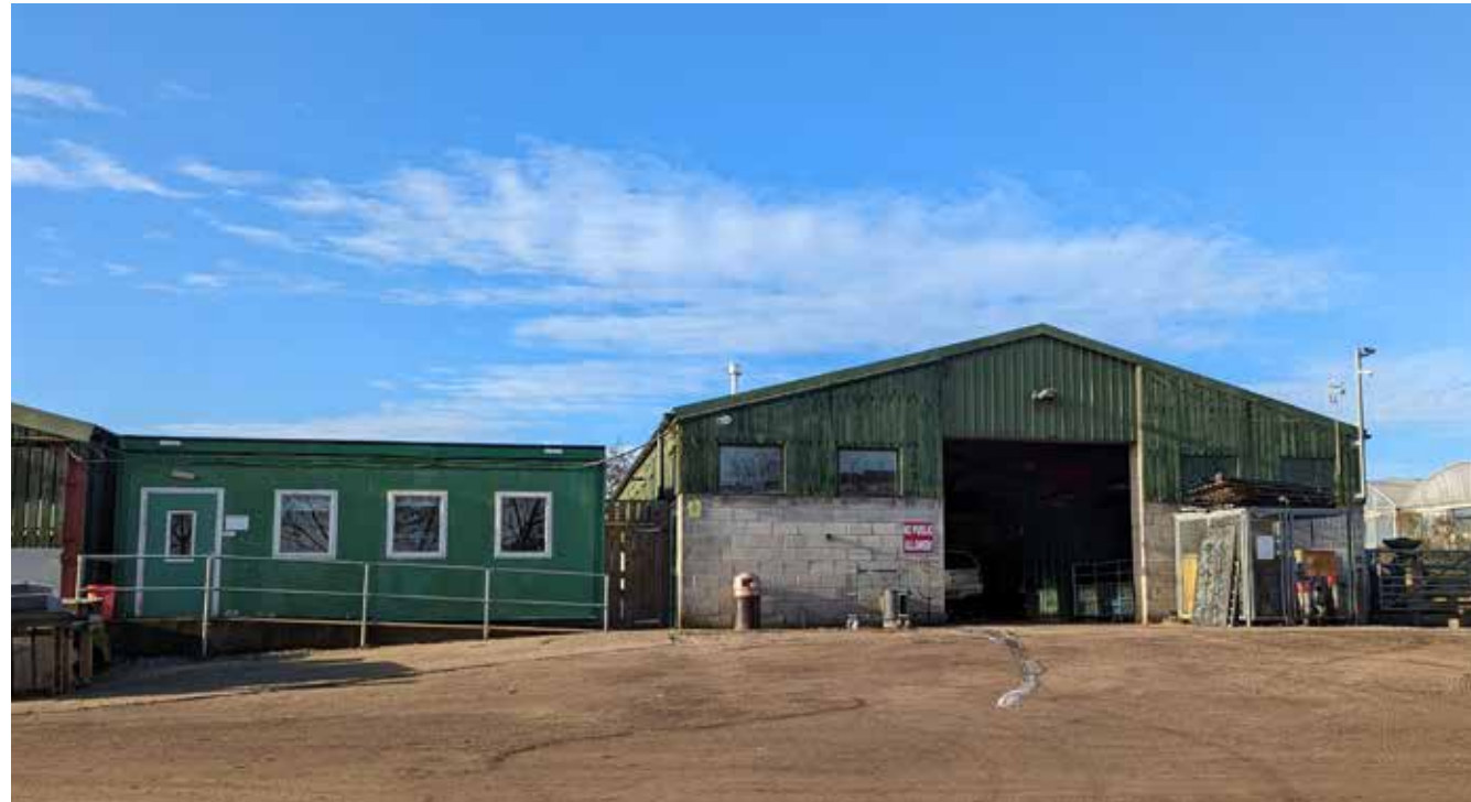
Photograph of East Elevation of existing Tractor Shed from east
