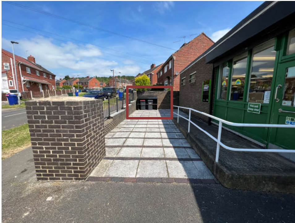
001 – ASHP compound location to be hidden behind existing bin store as highlighted
