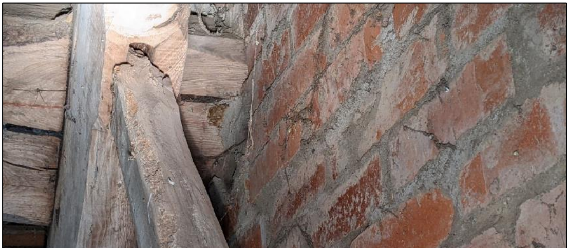
Plate 8. Open mortice joint in king-post truss in B2
