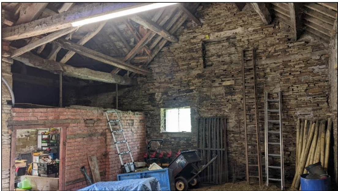
Plate 8. Open mortice joint in king-post truss in B2
