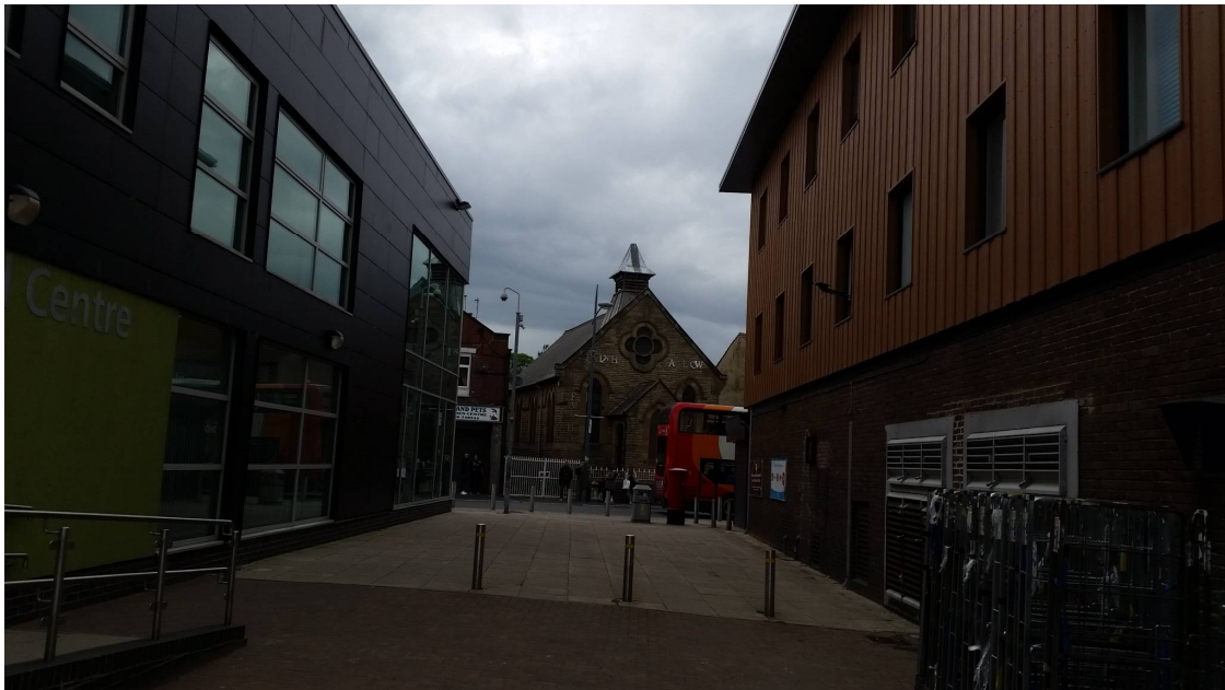
Picture 1: The building to the right is Former Council Offices . This measurement location is labelled ML2.
