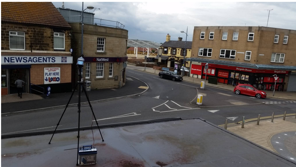
Picture 2: Measurements at the first floor level of Former Council Offices facing high street. This measurement location is labelled ML1.
